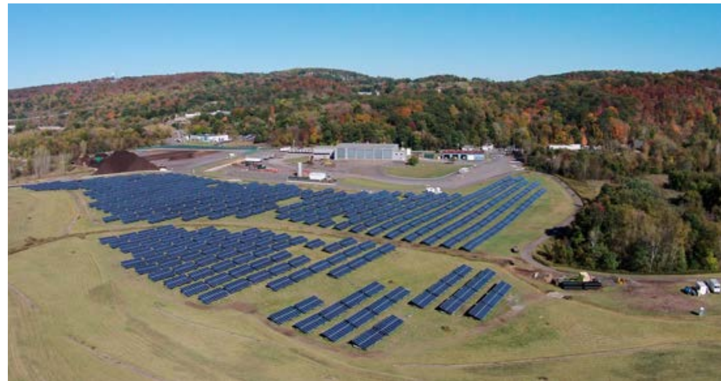
SOLAR FIELD ON MUNICIPAL LANDFILL, TOWN OF CLARKSTOWN (TOWN OF CLARKSTOWN)
